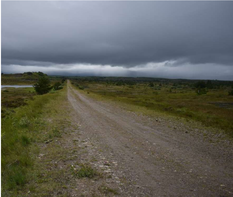
Figure 10.10 Access track of north L Dahybaun
